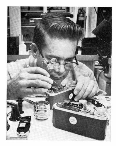
CAMERAS, timers, and mechanical indicators are typical repair jobs for Orval Talley and the other instrument technicians.
